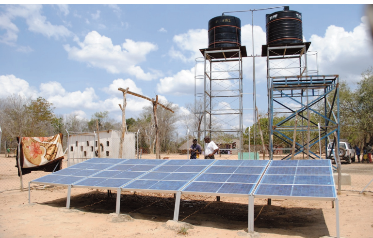
Image 3 and 4: Mozambique: Solar water pumping; Community solar battery charger
