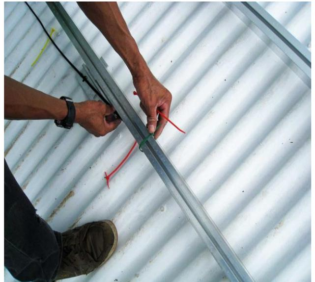
Temporarily tying the wiring to the rails
