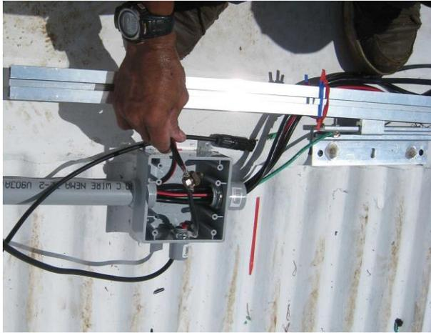
Completing the wiring in the main junction box
