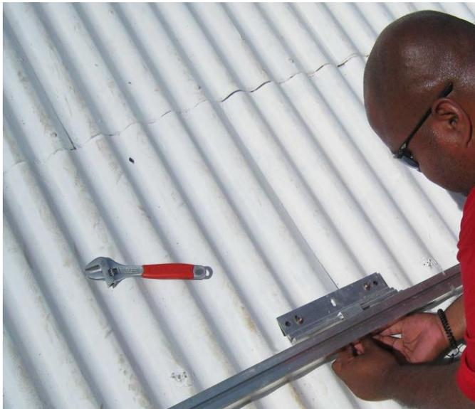
Fastening the rails to the roof
