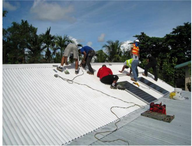
Laying out the panel attachment rails
