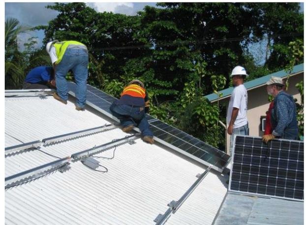
Mounting the panels on the rails
