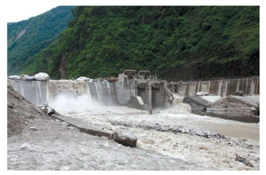
The Bhote Koshi hydropower 45 MW **Nepal** damaged by a flood. The Dig Tsho GLOF washed away a new hydropower plant in **Bhutan**
