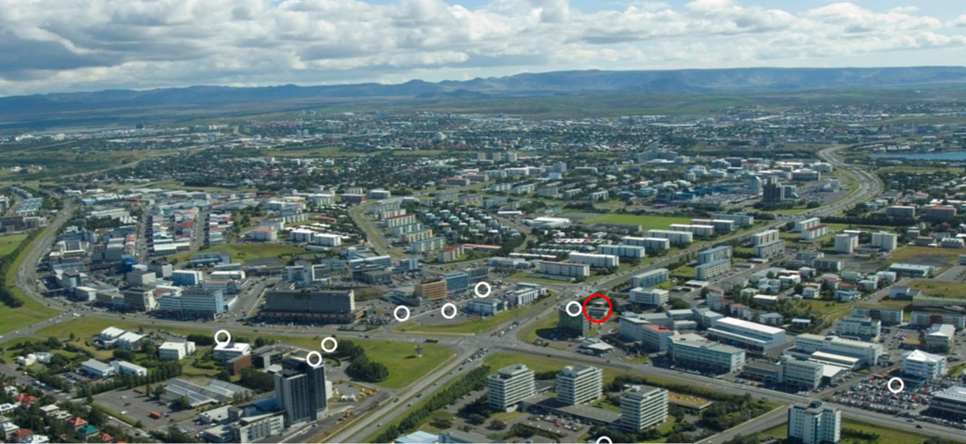
Reykjavik geothermal wells for district heating in the city
