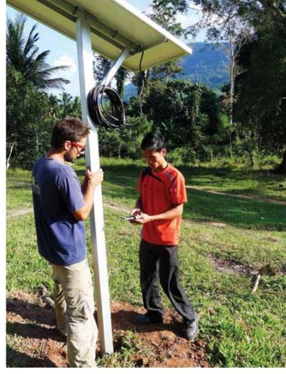
nstallation and orientation of a solar PV panel (ARE)
