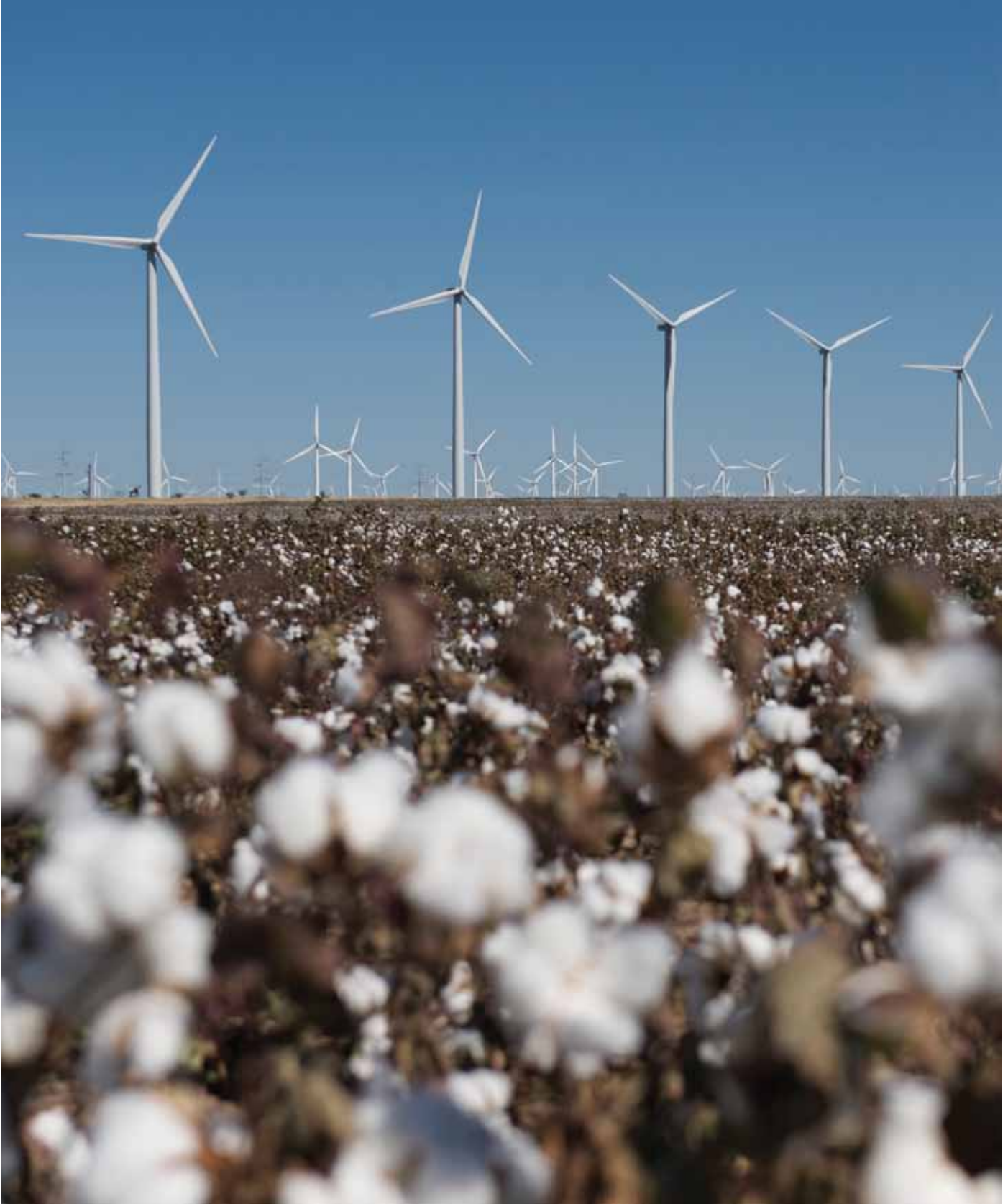
Horse Hollow, Texas, USA ©Wind Power Works
